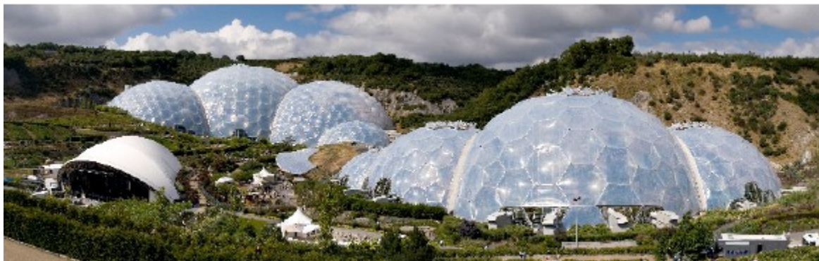
Figure 2: Eden Project in the United Kingdom
