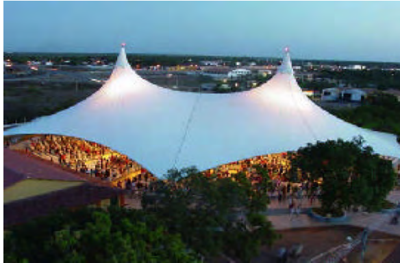
Fig. 2: A large membrane roof for the Baptist Church of Fortaleza (Pauletti et al., 2003)
