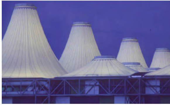
Fig. 1: The first extension of the park of expositions of Bordeaux-Lake (Société Bordelaise D'architecture, 1990)
