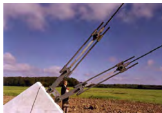
Fig. 15: Guy attachment to foundation with tension system
