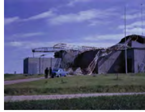
Fig. 18: 200 m mast in Sweden after insulator has broken, since lightning lit the oil in an insulator
