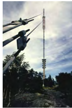
Fig. 14: The parabolas are fixed to the stiff concrete tower
