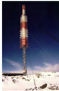
Fig. 13: Some masts are so heavily equipped with antennas so the wind resistance of the structure itself is not so important
