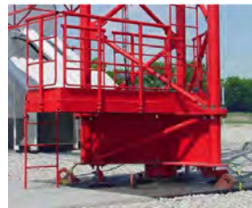
Fig. 16: Mast base foundation with pinned mast bearing
