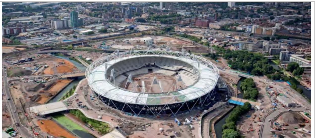
The London 2012 Olympic Stadium copyright Olympic Delivery Authority
