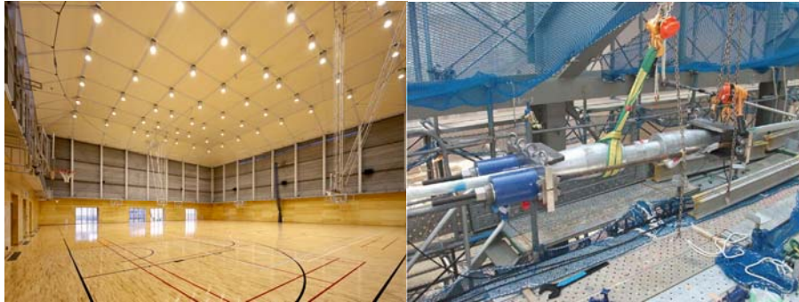
Figure 6: Interior of the Gymnasium and Prestress introduction
