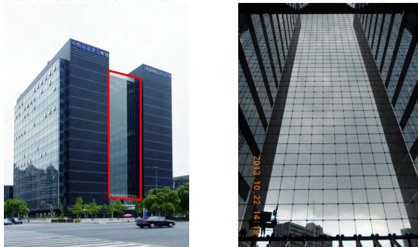
Figure 1: Shanghai Lujiazui Diamond Tower and its monolayer cable nets
